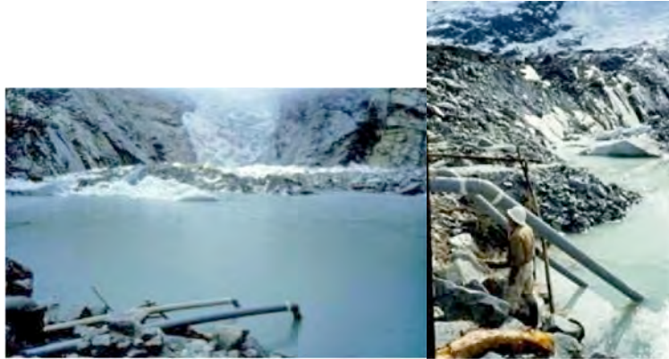
The initial siphoning process to lower the water level of Lake 513 in the late 1980s. Siphoning was an interim measure until funding was received for construction of the tunnel. Photos: César Portocarrero
