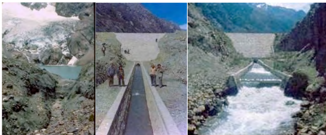
Constructing the Shallap Lake safety dam and water channel in 1973 and the completed work in 1974. Photos: César Portocarrero
